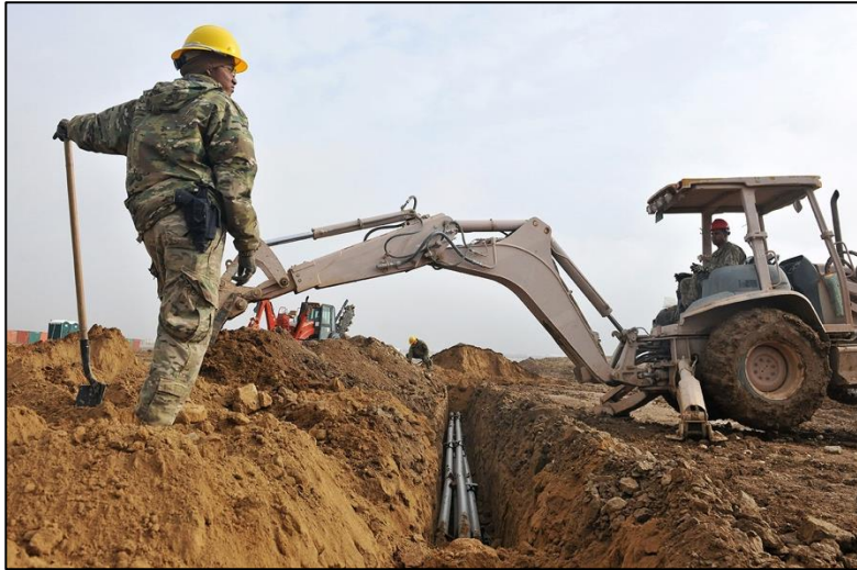
Figure 2-3. Reference photograph of manual and mechanical earthworks 10
