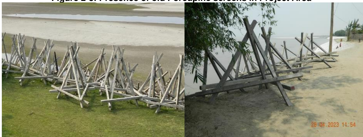
Figure 2-8: Presence of old Porcupine screens in Project Area 14
