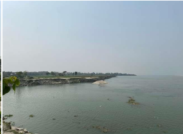
View of proposed site Makadhuj Spur to Faturi. No 1
