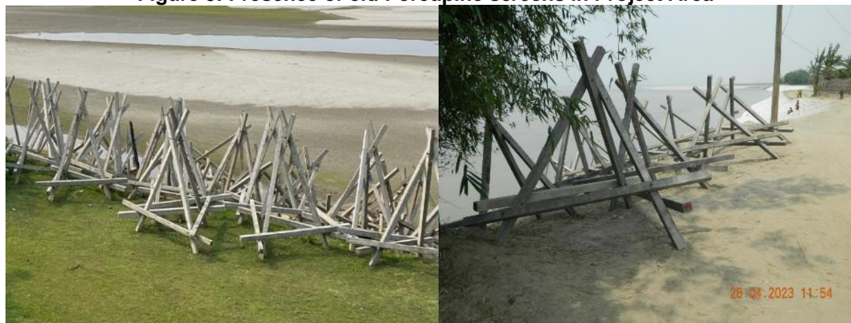
Figure 3: Presence of old Porcupine screens in Project Area 80
