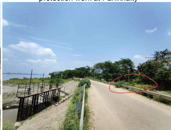
Proposed site for construction of Pumphouse Kalbhog channel at Palasbari
