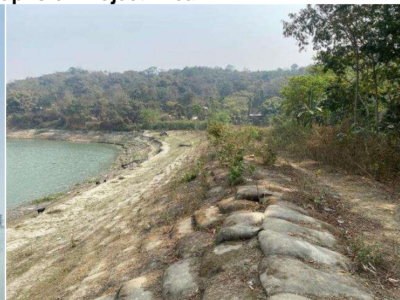
Upstream/downstream AE & FP work under AIFRERMIP Tranche II at Dakhala Kalitapara
