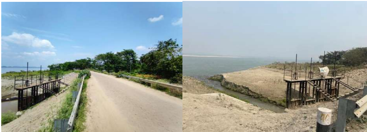
Figure 2-12: Sluice gate constructed at Palasbari under AFRIEMP
