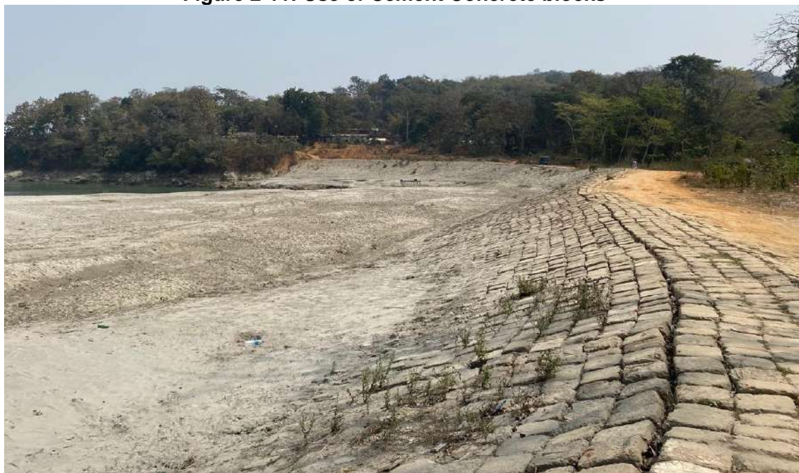
Figure 2-11: Use of Cement Concrete blocks
