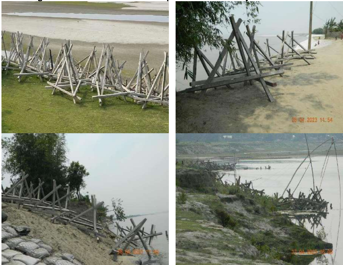
Figure 2-9: Presence of old Porcupine screens in Project Area 14
