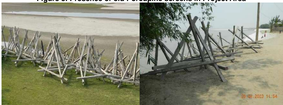
Figure 3: Presence of old Porcupine screens in Project Area 97
