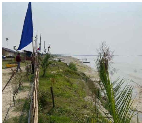
Proposed site for anti-erosion and flood protection adjacent to a Resort Chaulkhowa
