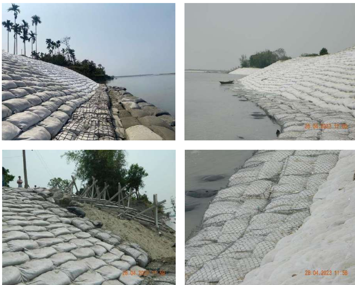
Figure 2-8: Use of Geo textile bags for Anti erosion works 13
