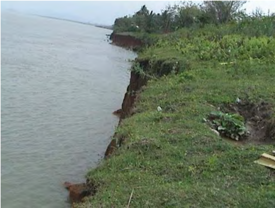
Plate 1: Erosion at Gumi
