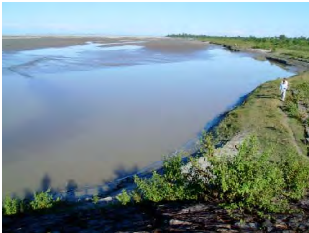
Plate 6: Riverbank Erosion upstream of Maijan Beel
