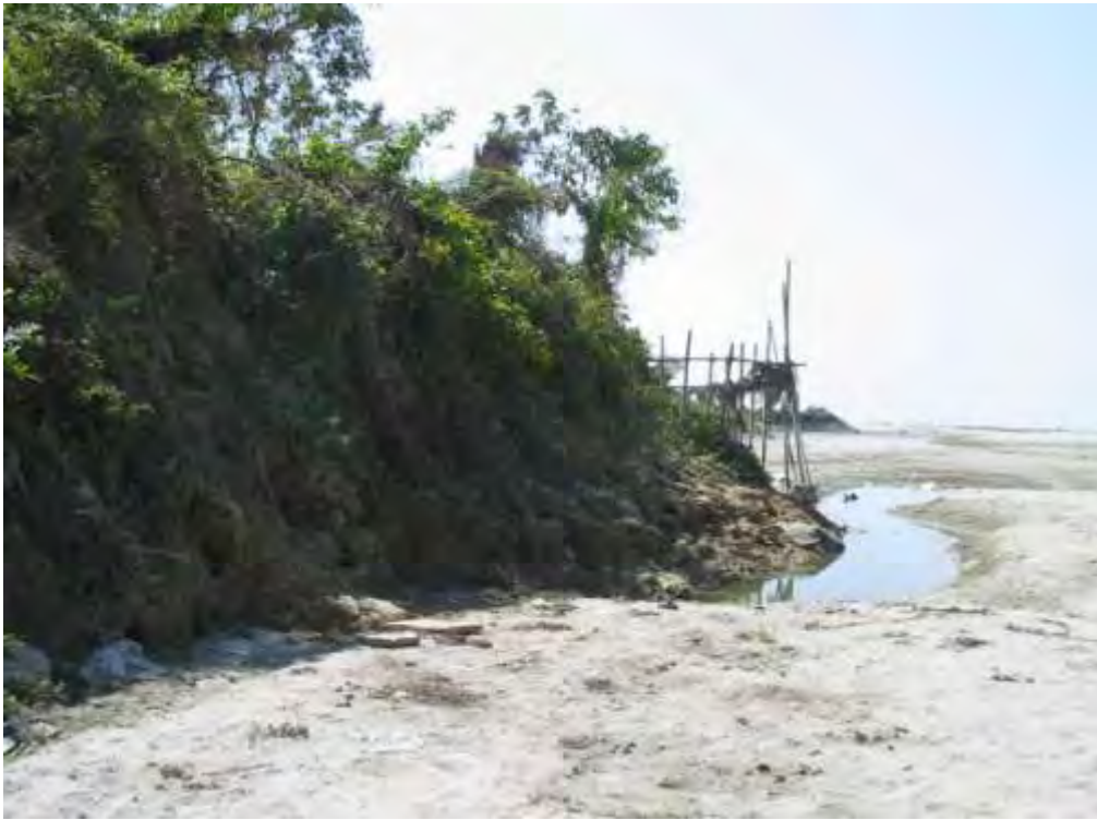
Plate 1: Erosion at Dibrugarh
