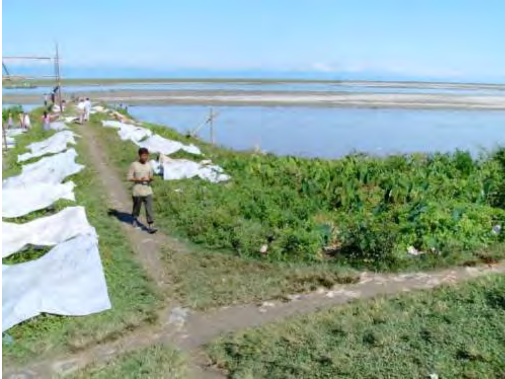
Plate 3: Existing Spur and Dibrugarh Town Protection Embankment
