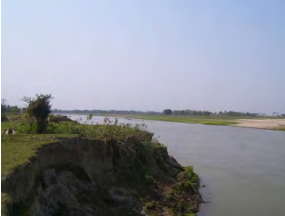
Plate 1: Erosion near Dhansirimukh
