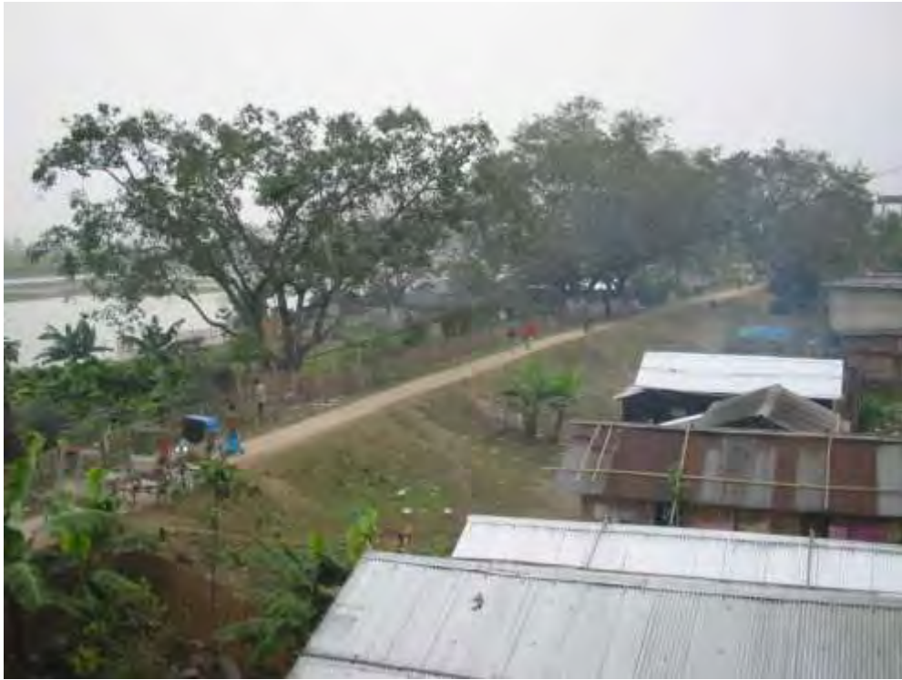
Plate 1: Existing Town Protection Embankment
