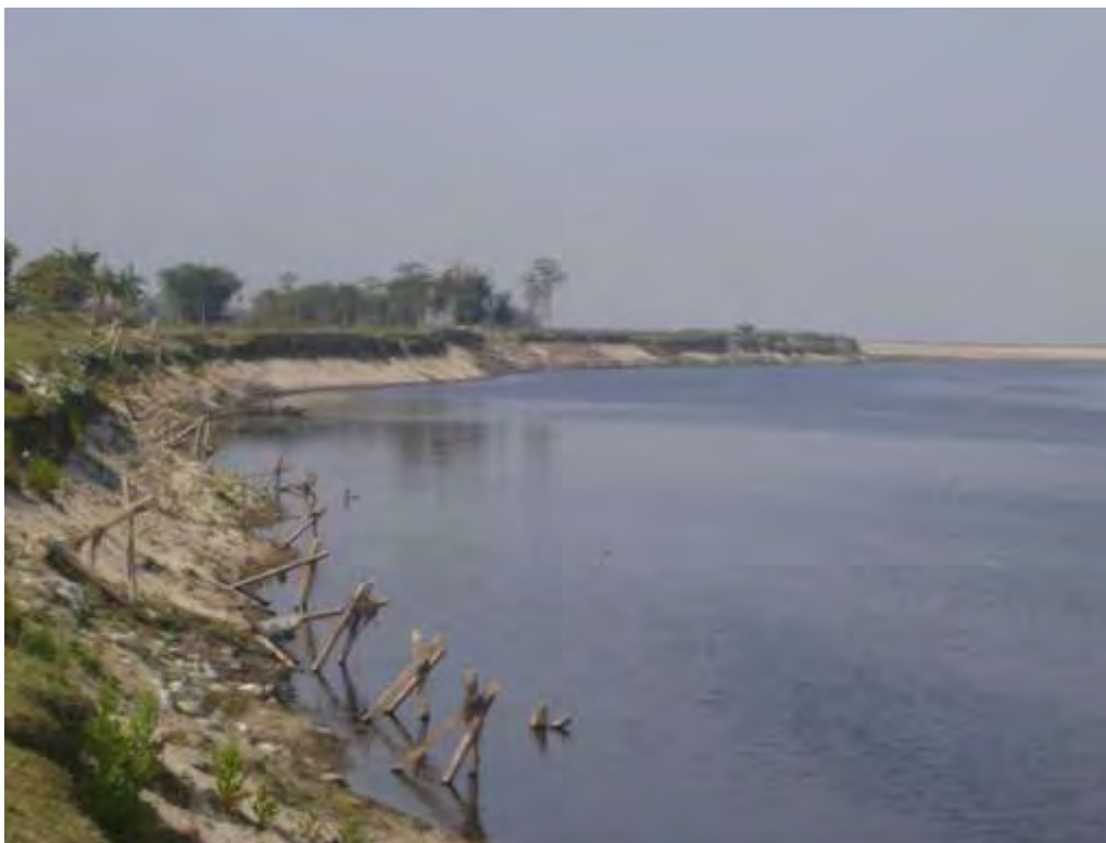
Plate 3: Riverbank Erosion (at Sakopara)
