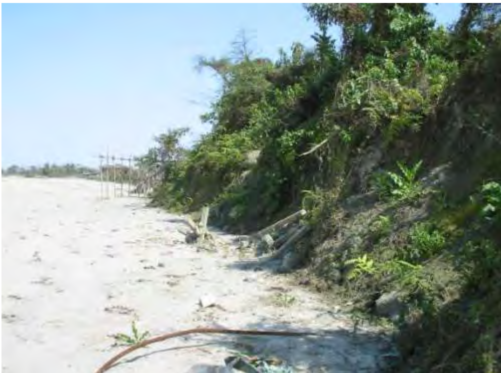
Plate 2: Erosion near Dibrugarh
