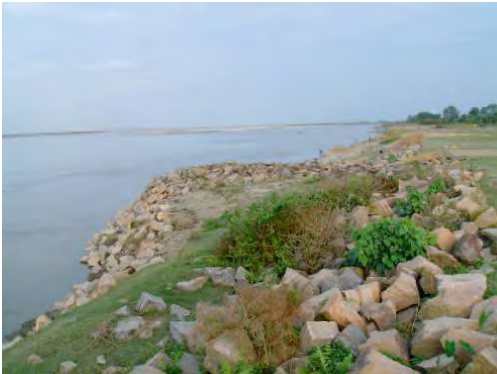
Plate 2: Existing Boulder Flow Deflector (near Gumi)
