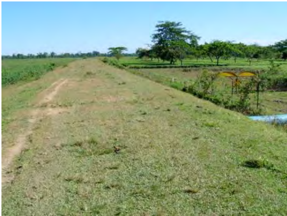
Plate 2: Existing Embankment along Maijan Beel
