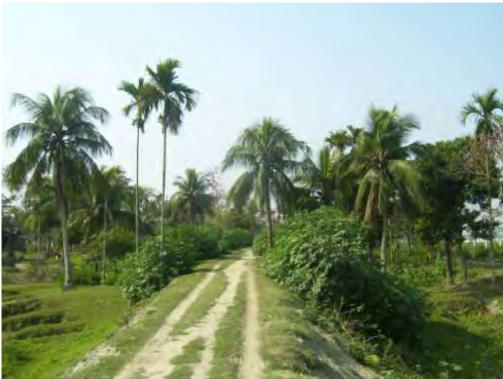
Plate 2: Existing Embankment along Kaziranga National Park Border (Right Side)
