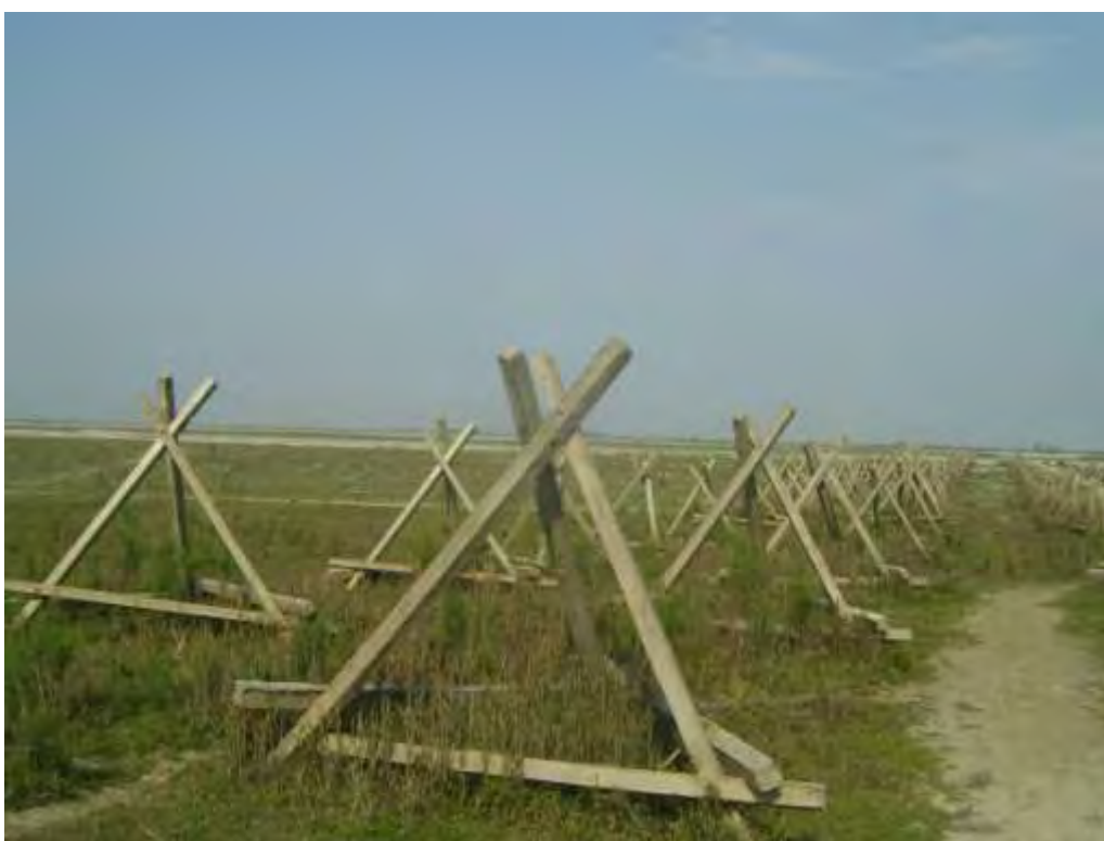
Plate 4: Porcupine Structure (Newly Placed)
